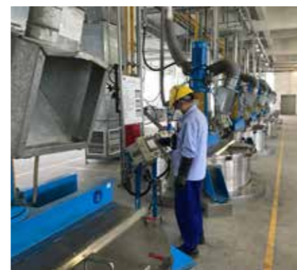
A technical personnel is doing daily maintenance of equipment.
