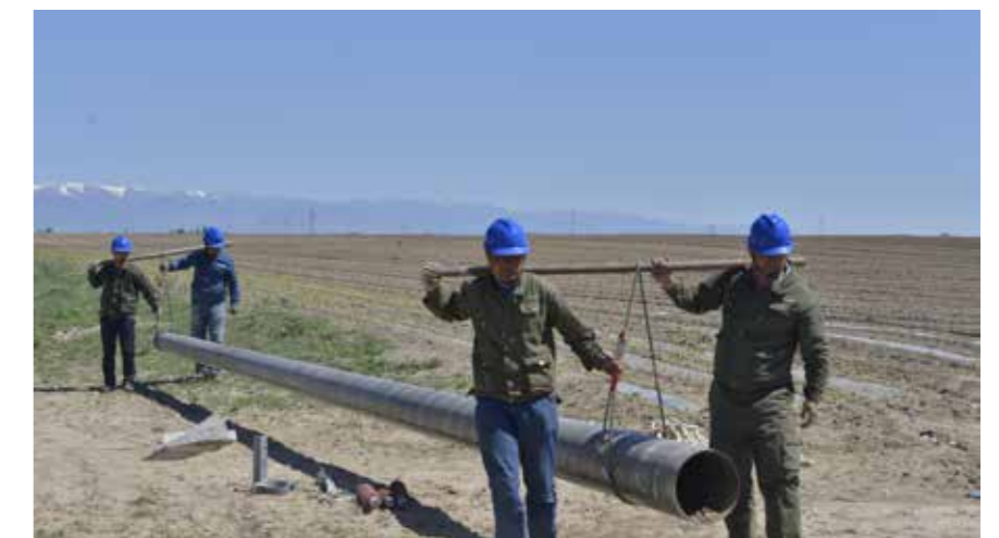
Weighting one-sixth of traditional poles, installation of composite utility poles can greatly save manpower.
